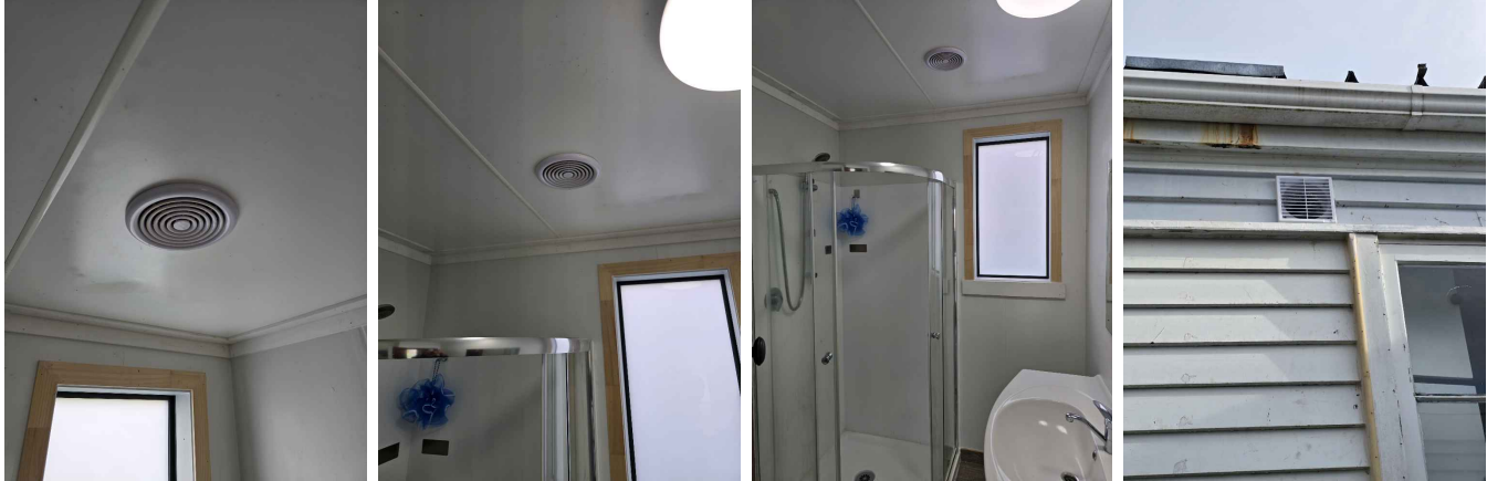
Pre-Existing Extraction Fan for Ventilation (Bathroom) Photo
