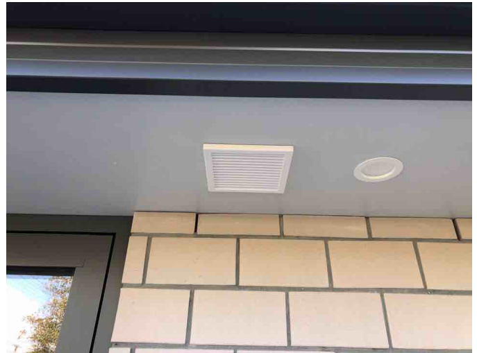
Vented to the exterior through soffit
