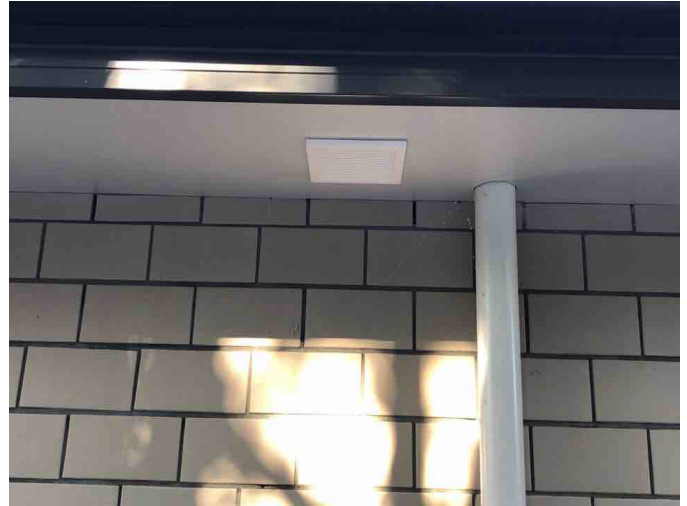
Vented to the exterior through soffit
